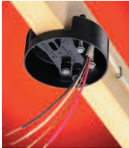
3 Pull NM cable through connector.
