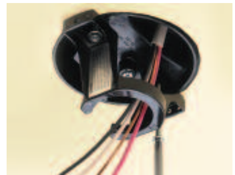
4 Remove two long, parked screws. Use to install bracket...
