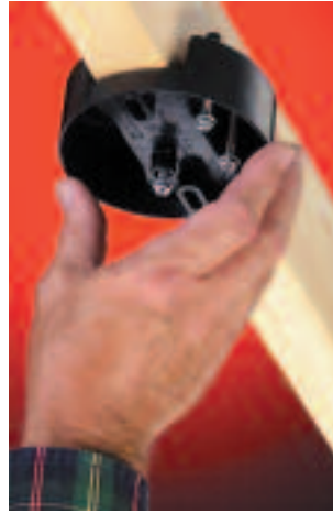
1 Press box onto joist.
